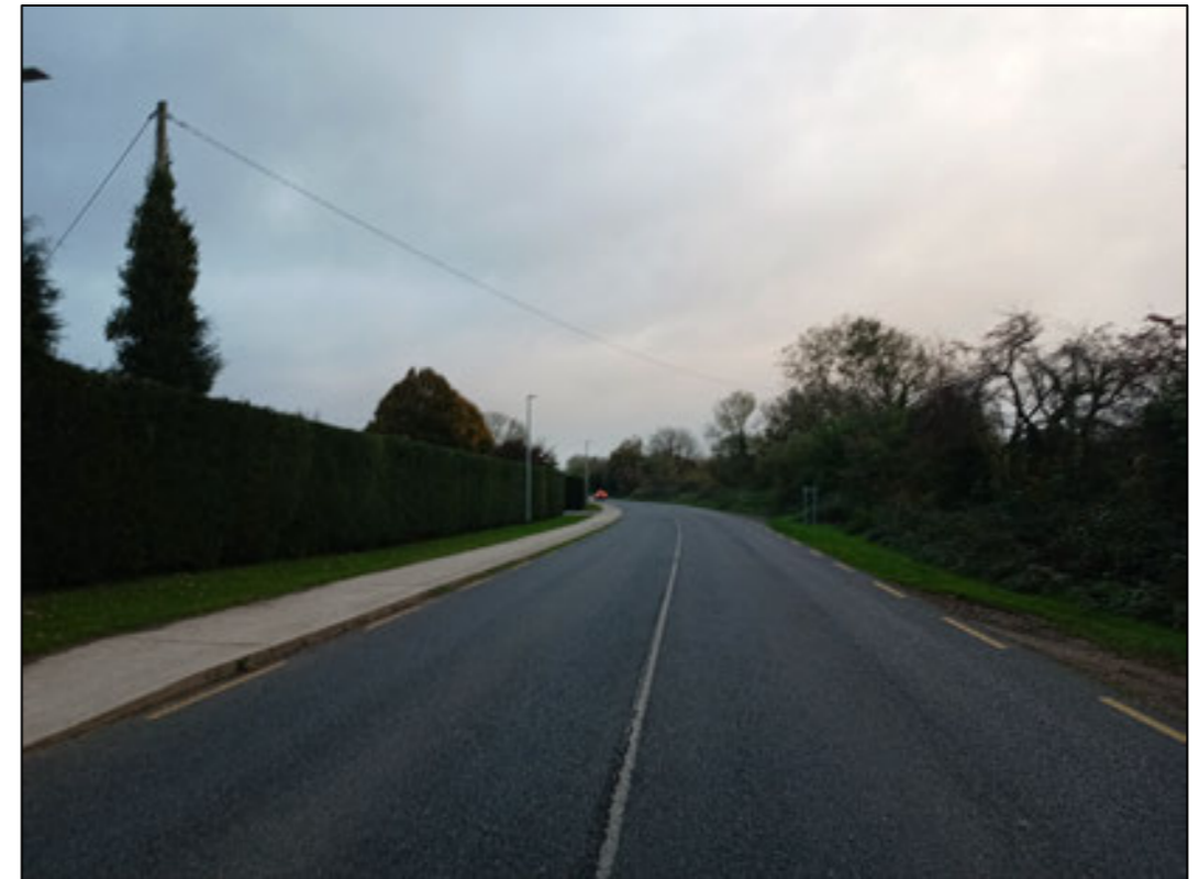
Plate 8: View of Carnew Road R725 from junction with proposed pedestrian/cycle path, facing northeast
