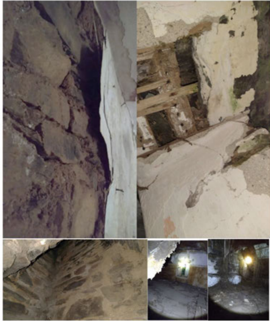
Wall plaster, window frames, chimney and checked for bats in September and March
